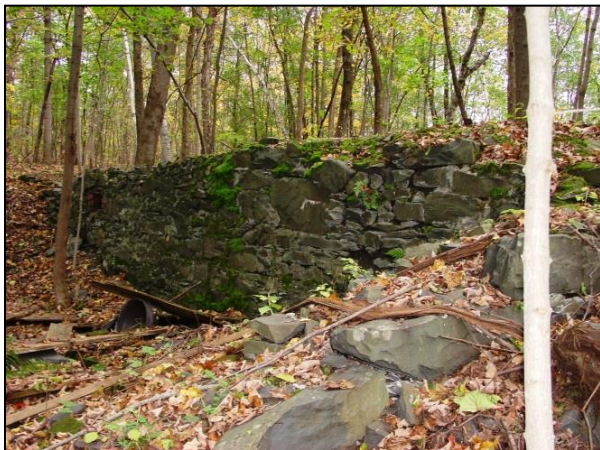
Photograph 67. View southeast showing the inside south wall of Feature H, the boiler house, with the west wall in the foreground.
