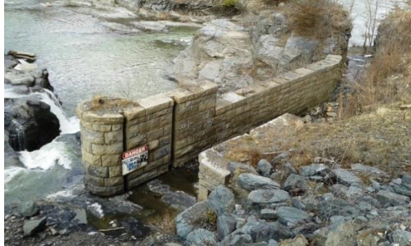
Photograph 56. View west from Mill Street showing remnants of the flume along the riverbank in 2017.
