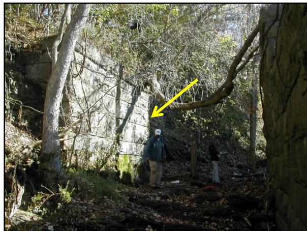
Photograph 57. View from inside the flume in 2008 showing the stone wall built against the slope. Vertical channels for a gate mechanism were present at its east end (yellow arrow).
