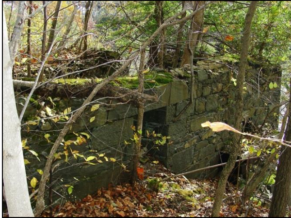
Photograph 66. View southeast of the exterior wall of Feature G, the machine shop. Note opening where line shafting passed from power system to the mill.
