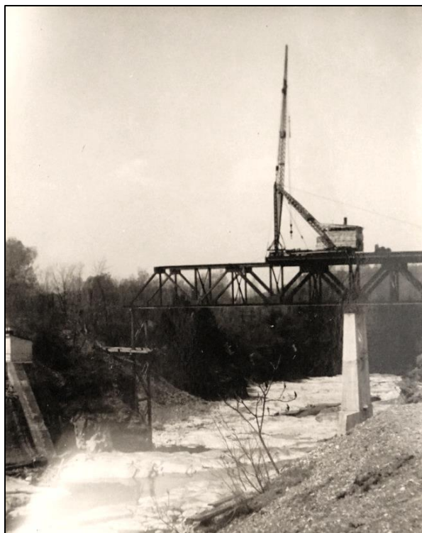
Figure 105. View of the truss being built out from pier 3 across the west side of the river channel. A crane is being used to lift truss members into place. Steel instead of timber falsework is used to support the truss due to heavy outflow from the hydroelectric dam (Courtesy of Schaghticoke Village Historian).
