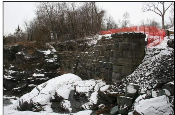
Photograph 58. View north showing remnants of the flume's outer wall after clearing for bridge construction in 2014.
