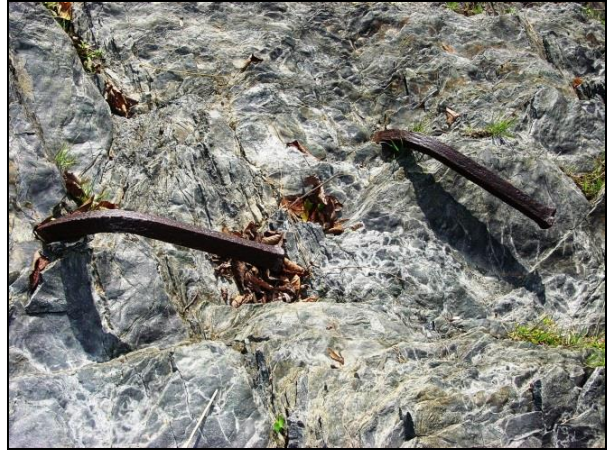
Photograph 68. View of metal bars imbedded in the riverbed where the wooden members of the north dam (Feature E) were held in place.
