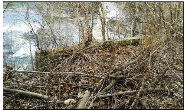
Photograph 74. View northwest of the poured concrete retaining wall feature at the top of the cliff in the Cable Flax Mill Site.
