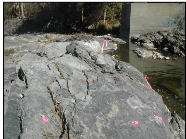
Photograph 59. View northeast beneath the bridge showing the locations of drill holes with metal rods (marked with pink tape) used to anchor the dam in the river bed.
