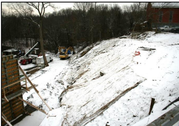
Photograph 81. View north of Mill Street during the new bridge construction.
