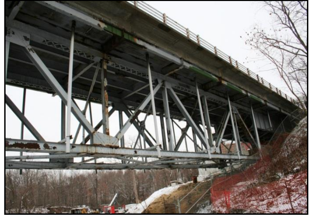
Photograph 82. View northwest near the 1941 bridge showing slope below the A. Briggs and Hart Estate Site protected to avoid damage from new bridge construction.
