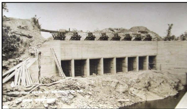
Photograph 9. Ca. 1908 power canal.
