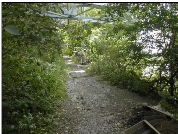
Photograph 72. View south showing the former alignment of Mill Street, just a gravel path at the time of testing. Note the underside of the Route 40 bridge.
