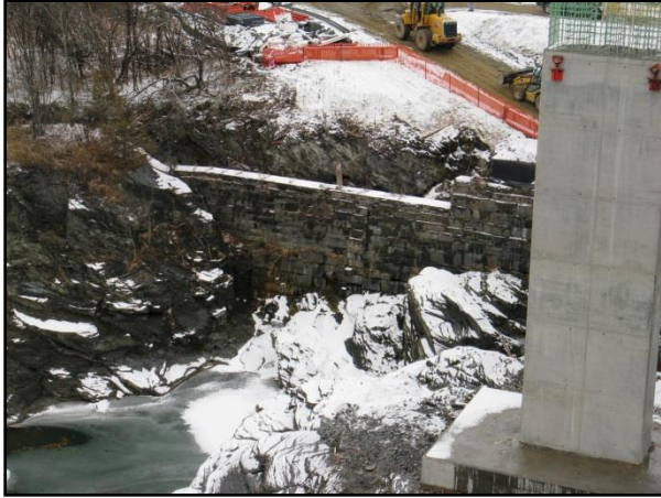
Photograph 79. View north of ca. 1830s stone flume associated with the Schaghticoke Woolen Mill, protected to avoid damage from new bridge construction.
