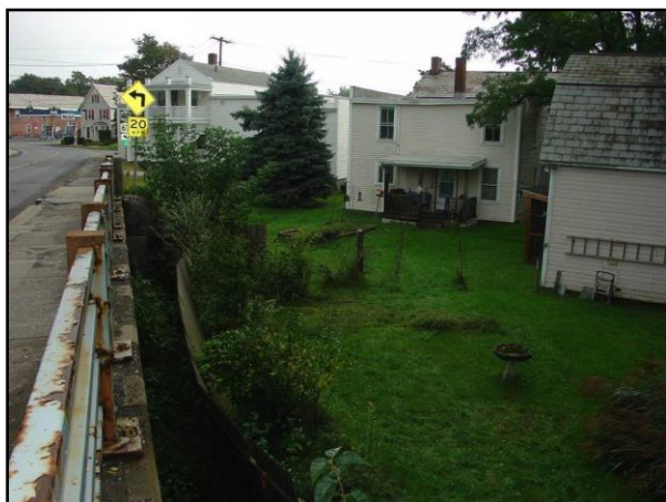
Photograph 43. Looking northeast at the rear yards of #177 Lower Main Street (P. Briggs Site foreground, right) and #173-175 Lower Main Street (Baker Block Site, background, left) along Route 40 at the northern end of the bridge.
