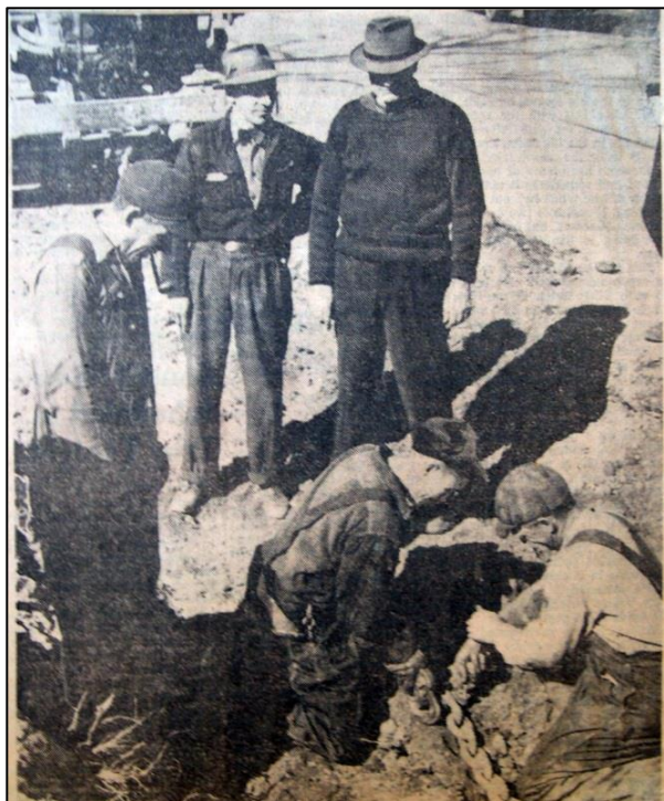
Figure 107. Photograph of Frank Antolick (left rear) and George Cummings, Schaghticoke water and street commissioner (right rear) overseeing the removal of a water pipe during the construction of the Route 40 bridge (Courtesy of Schaghticoke Village Historian).
