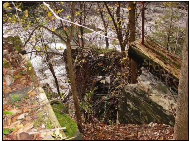
Photograph 65. View of Feature G, the machine shop (left), Feature F, the wheel house (center foreground), and Feature D, the flume house (background). Note wooden components still present in the upper portion of the wheel house.
