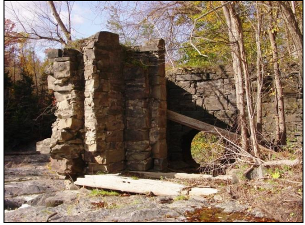
Photograph 63. Close-up of the remnants of the flume house (Feature D) and the round opening at rear for a penstock or pipe into the wheel house (Feature F).
