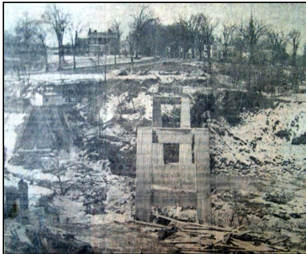
Photograph 11. December 1940 bridge construction showing most of the A. Briggs and Co. Housing Site. View is southwest. (TR Dec. 10, 1940: Page 6).
