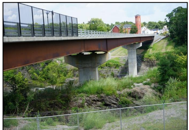
Photograph 83. View north of the new Schaghticoke Bridge after removal of the old bridge.
