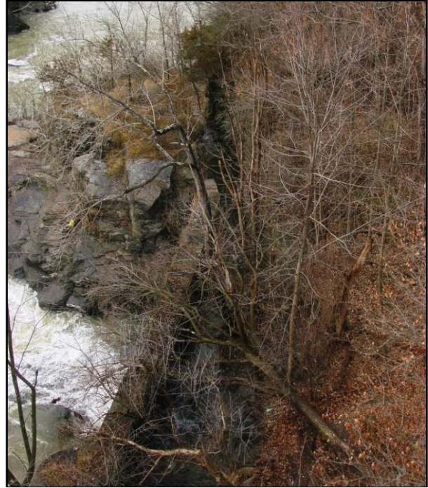
Photograph 53. View north showing remnants of a flume along the river bank.
