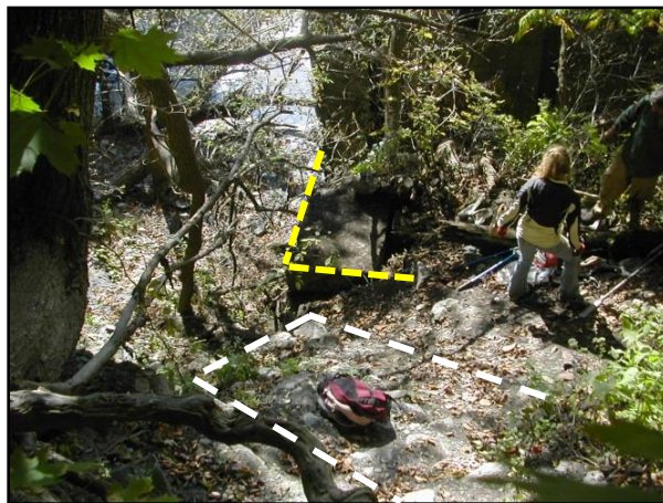
Photograph 55. View west showing evidence of the building foundation (white dashed line) along the steep slope on the northern bank of the river. The eastern end of the flume's northern wall is outlined in yellow.
